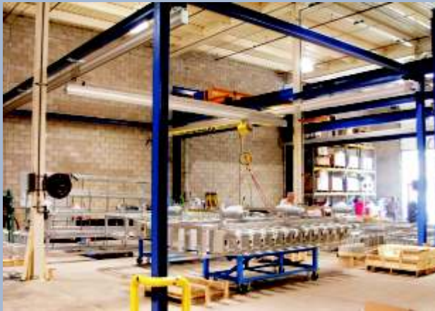
A builder of components for the power transmission industry utilizes a conventional freestanding single girder system to safely handle high value loads.
